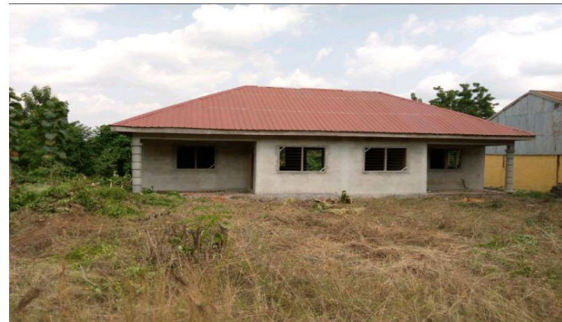
B. Construction of Tsito Town Council Office at Tsito
